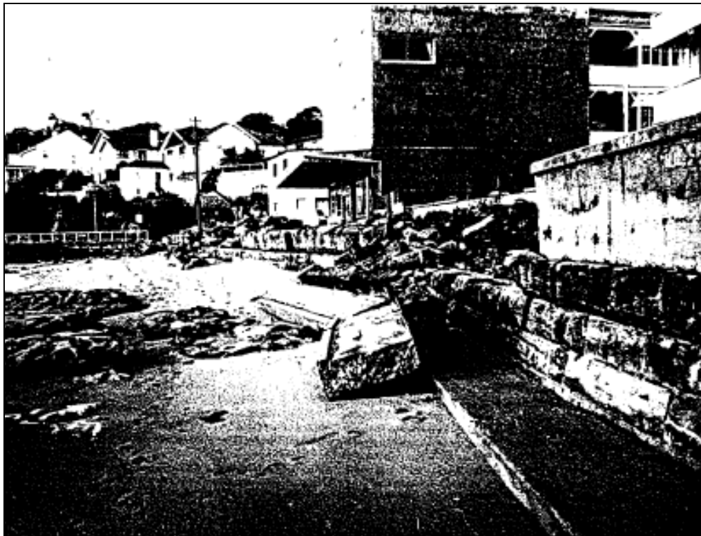
Photo 1.9 Damage to upper courses of blockwork and coping at Fairy Bower seawall caused by the May/June 1974 storms
