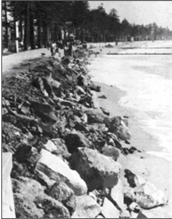
Photo 1.4 Emergency rock protection at South Steyne in about 1967-1968
