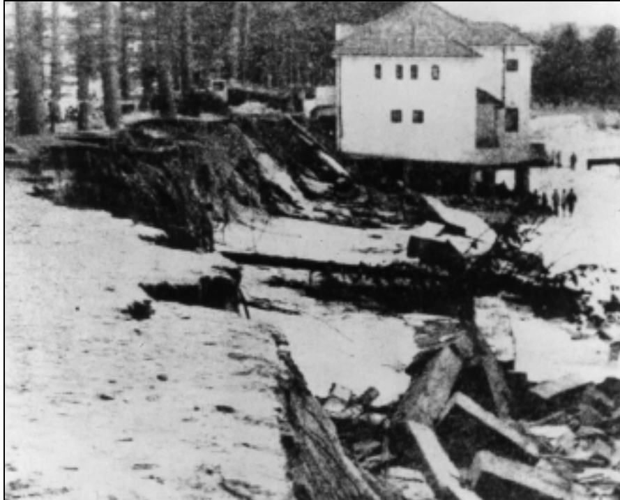
Photo 1.1 Beach erosion and seawall, promenade and landscape damage looking north towards North Steyne SLSC, 1950. Note piling under North Steyne SLSC.
