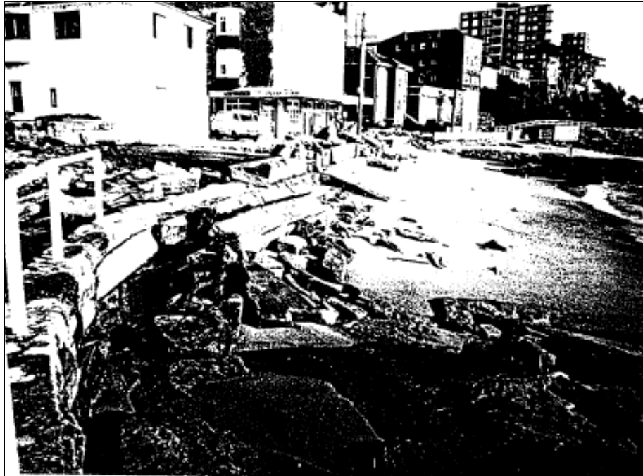
Photo 1.8 Damage to upper courses of blockwork and coping at Fairy Bower seawall caused by the May/June 1974 storms
