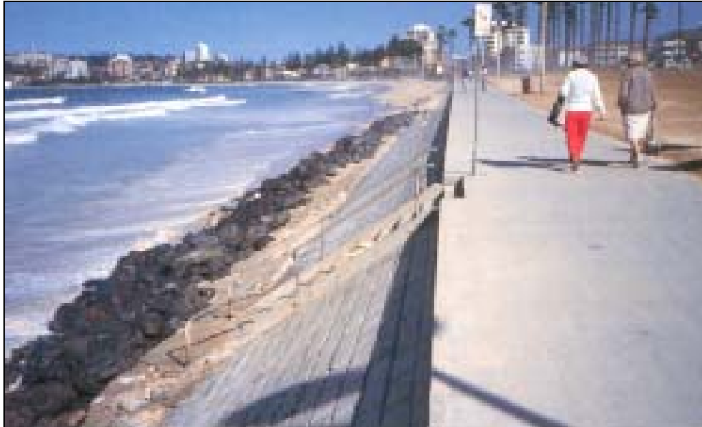
Photo 1.10 Exposure of rock protection at Queenscliff in approximately 1986
