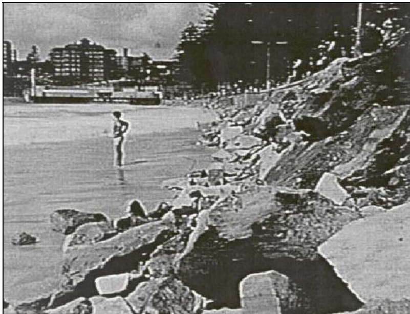
Photo 1.5 Emergency rock protection at South Steyne, 1974
