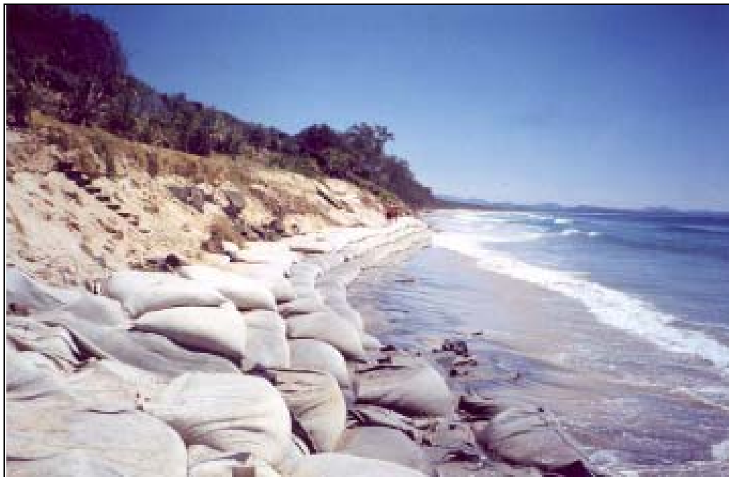
Photo 4.1 Geobags at Belongil Beach Byron Bay, NSW (after WRL, 2003)
